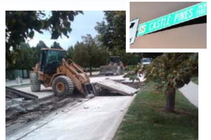
Initial road construction has begun on westbound Castle Pines Parkway
